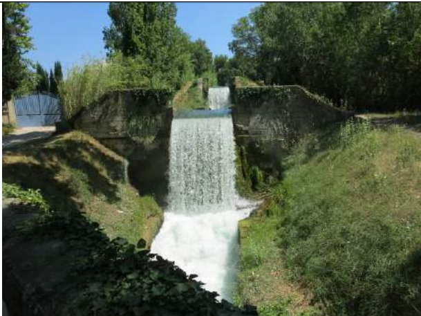
Figure 45: Main irrigation Channel at St Remy
