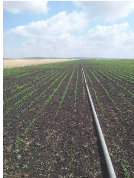
Figure 8: Irrigation pipes laid out
